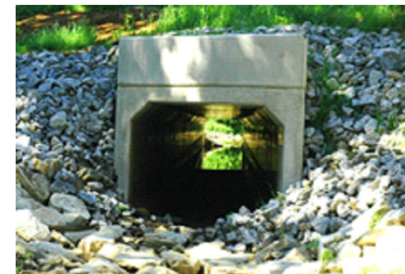
CULVERT OUTLET @ DISCHARGE POINT
